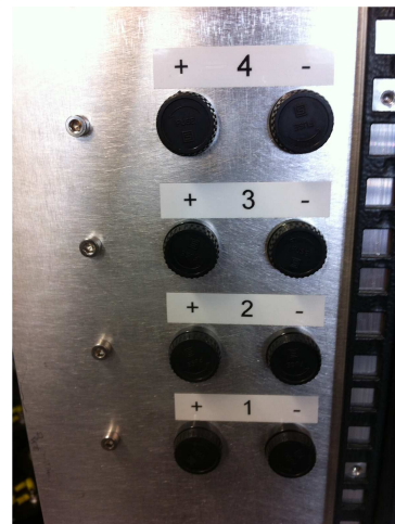
Fig 8: The fuses inside the generator
